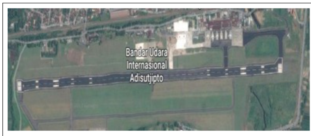
393 394 Fig. A3. Map of Runway in Adisutjipto International Airport -AIA (taken from (Najamudin, 2017)).
